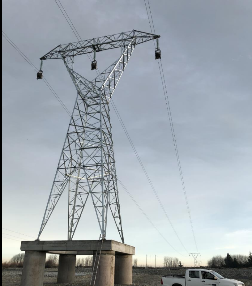
New tower on new river foundation
