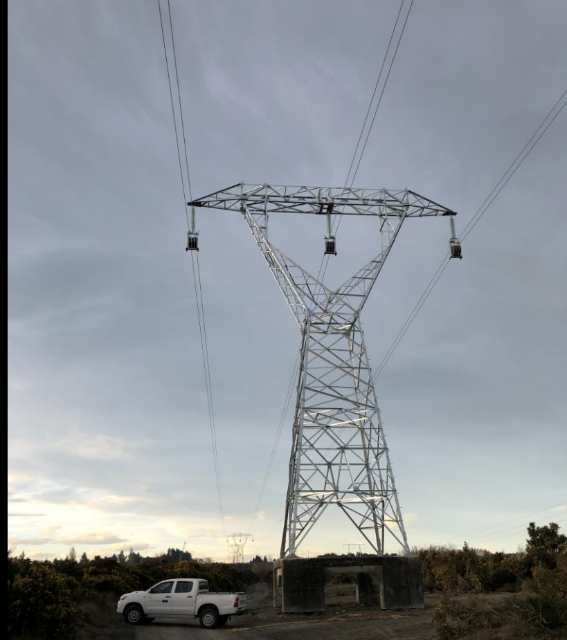
New tower on existing river foundation
