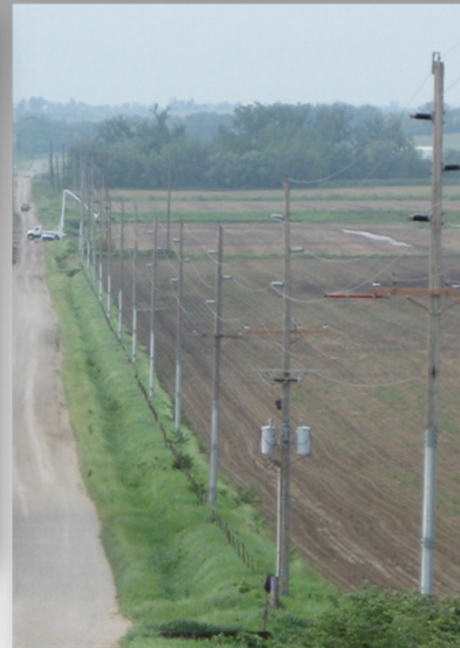
Entire section reinforced
