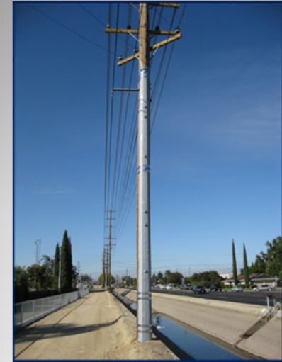
Capacity upgrades ET truss
