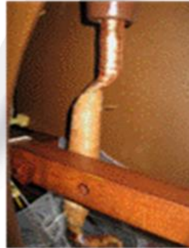
Enlarged view of lead wrapped with insulating paper
